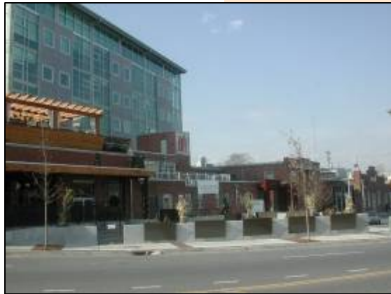
Street-level retail in the Gulch is designed to generate pedestrian activity.
