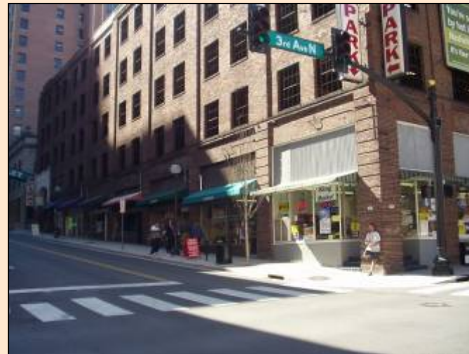
This garage on Church Street illustrates that active ground-level spaces can be incorporated into the design of parking structures.
