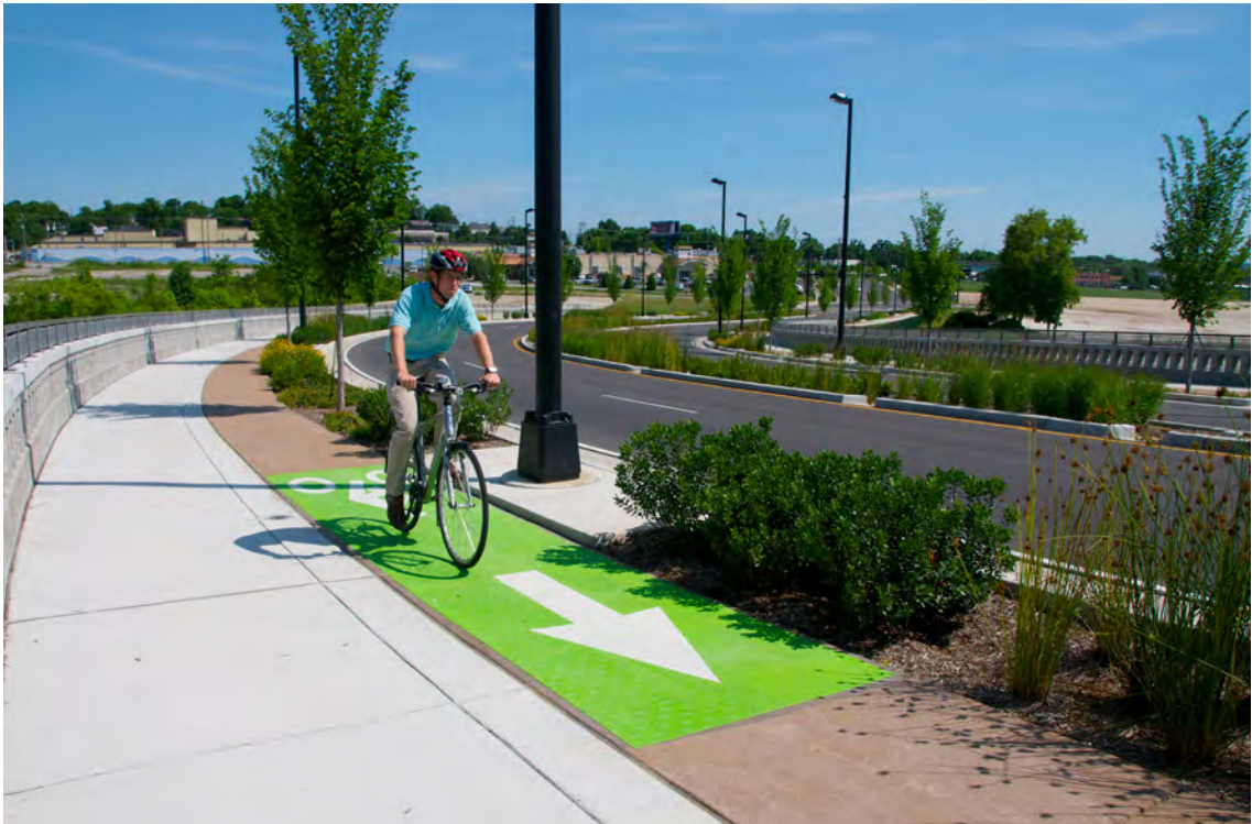
Cycle track is clearly defined through the change of hardscape materials
