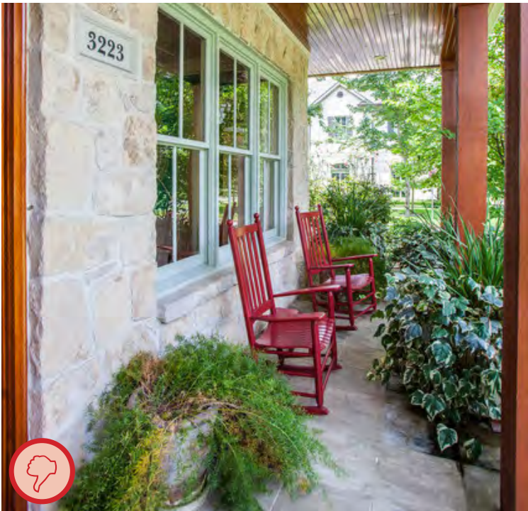
Inappropriate: Porch depth is not functional
