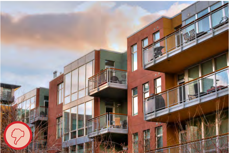
Inappropriate: EIFS should not be provided near accessible or “touchable” areas such as exterior balconies
