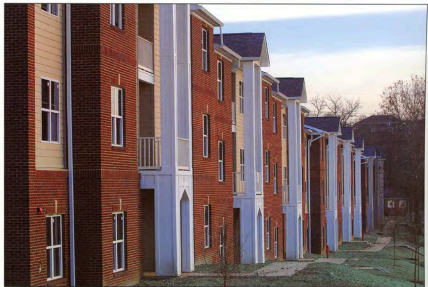
Construction of the new East River Place Apartments, which provide housing to low- to moderate-income Nashvillians, was aided with community development funding.
