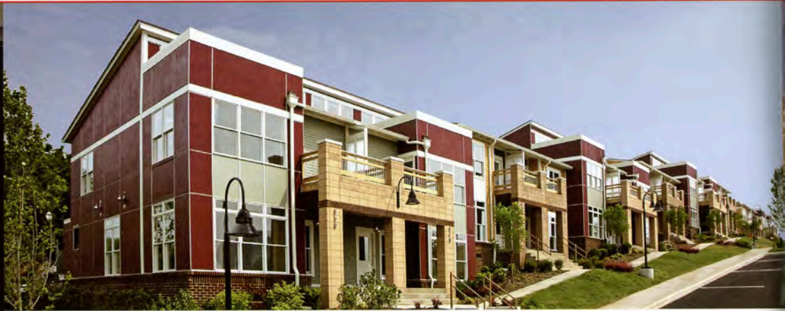
(above) Ireland Street Townhomes, built by Affordable Housing Resources with assistance from MDHA, offer views of the downtown skyline from the Hope Gardens neighborhood.
