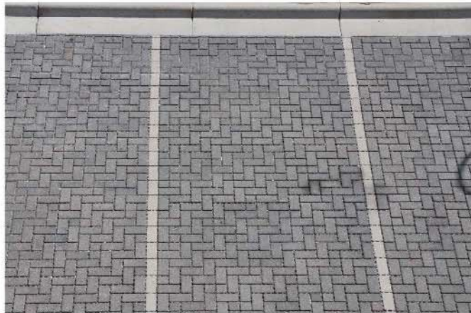
Pervious pavers are used in parking stalls to reduce site stormwater runoff.
