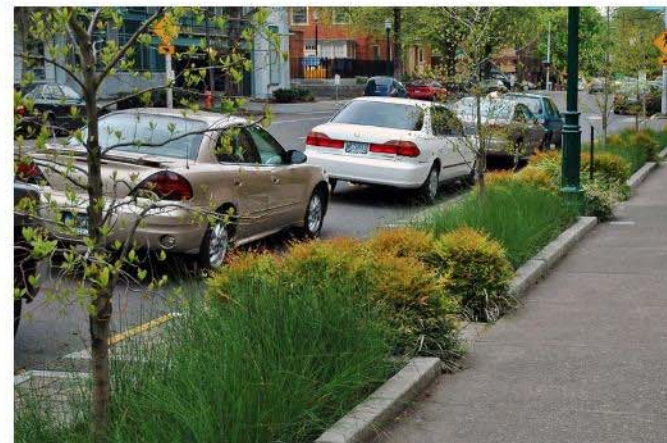
Curb inlets direct stormwater into bioretention facilities located within the "Furnishing Zone".
