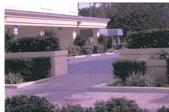
Low walls, when used in combination with plantings, are an effective screening element.
