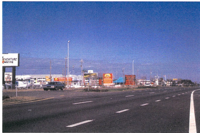
This generic strip commercial development is dominated by signage and parking. Designed specially for automobiles, it is inappropriate for the Gateway Subdistrict.
