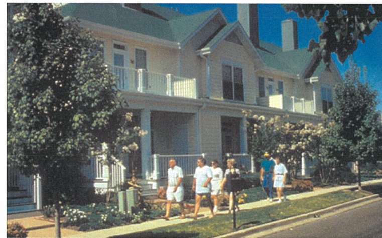
Rooflines, projecting bays, recesses, and porches can be combined to break up the massing of multi-family buildings
