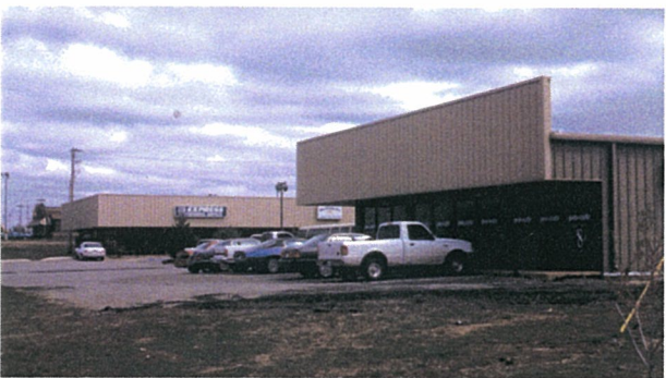
This overhanging "fascia" type roof is inappropriate for the Woodland Street Subdistrict.
