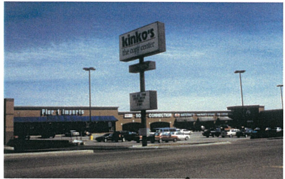
Free-standing signs that dwarf their associated buildings are prohibited.
