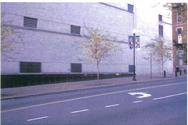
This building's bare facade does not promote pedestrian activity. With no windows, entries, or canopies on the street, this building is inappropriate for Woodland Street.
