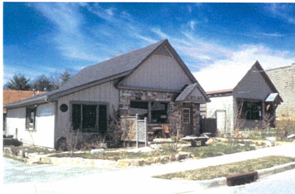
The applied false stone on the exterior and the cluttered appearance of the yard make this building inappropriate for the Residential Subdistrict.
