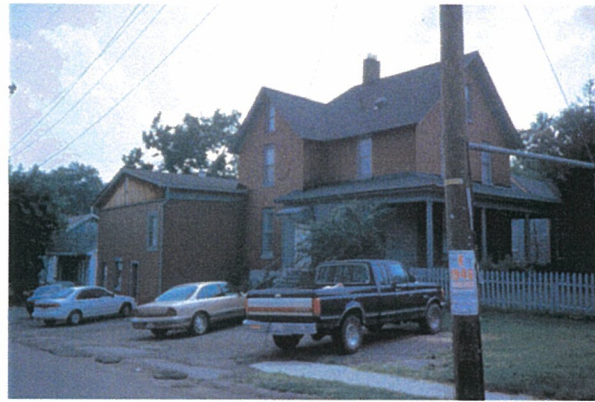
Front parking detracts from the streetscape and interrupts the sidewalk.
