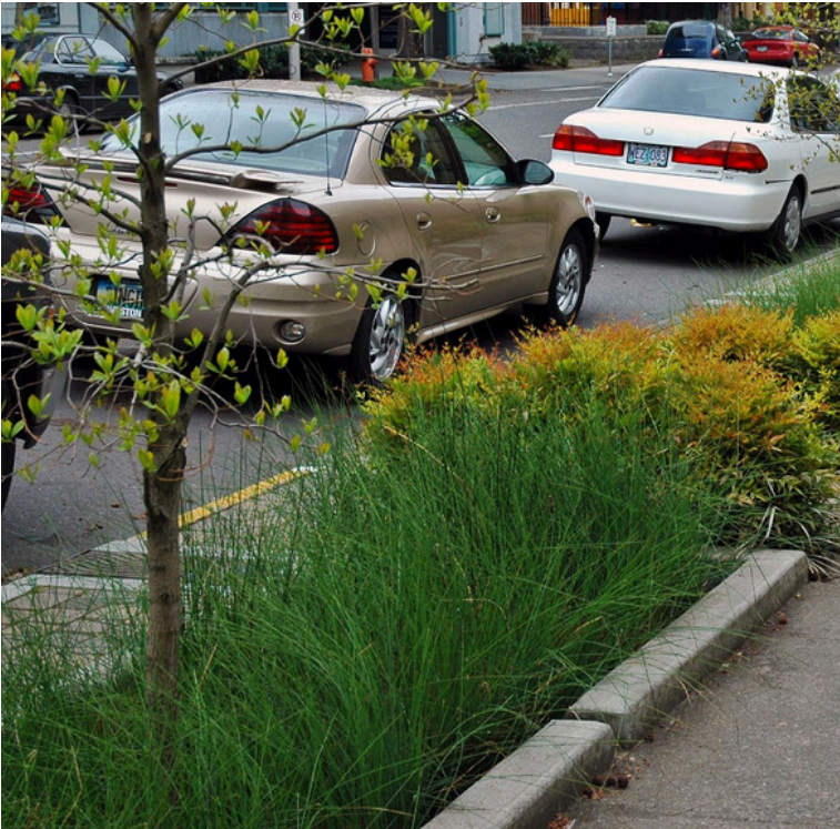
Curb inlets direct stormwater into bioretention facilities located within the “Furnishing Zone”
